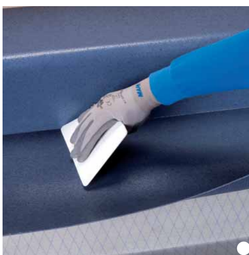
Massaging the PVC after applying Mapecoat
