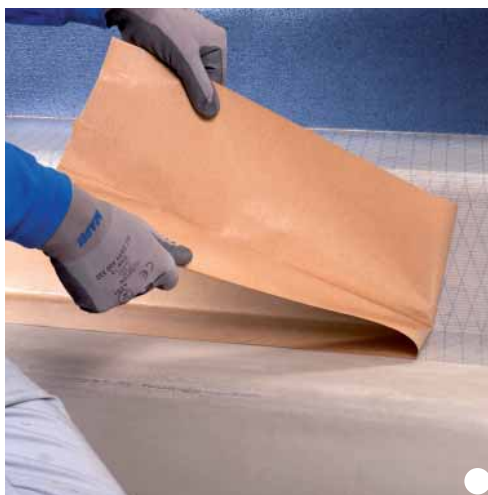
Removal of the protective coating
