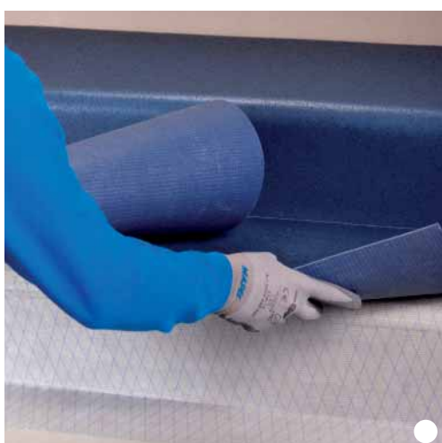
Application of PVC on steps using Mapecontact
